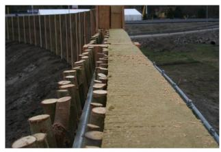
Birds eye view of barrier top showing woven panels, the noise absorbent core, and mesh panel.
