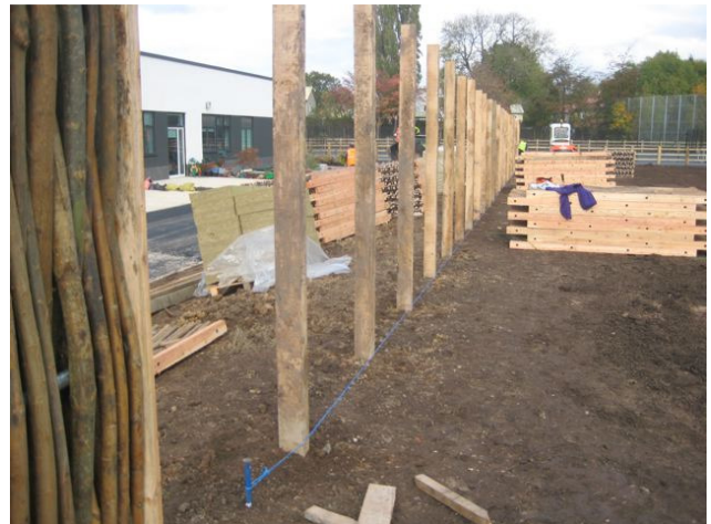
Hardwood posts installed and first side panels attached
