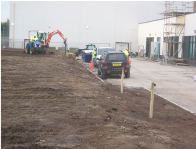
Positioned at top of bank, to maintain maximum acoustic screening
