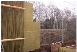
This barrier is constructed with one side living willow, a sound absorbing core, and the other side is metal security fencing.
