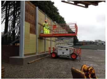
Noise absorbing RockDelta core being put into place.
