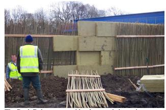
The Rock Delta core provides the sound absorption, giving an 11db reduction in noise.
