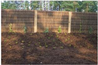
The 2m high Green Barrier erected on a 1.5m soil bund, softening the appearance and providing additional height to the acoustic screen.
