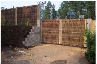
Sound attenuating gates incorporated, using the same high quality soundproofing material as the barrier.
