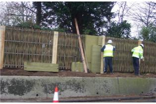
The acoustic insulation being installed and the facing panels erected.
