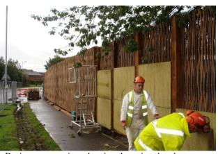
During construction, showing the noise absorbent core inserted between the woven willow panels.
