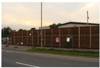
Finishing off the installation of the acoustic Green Barrier<sup>TM</sup>.
